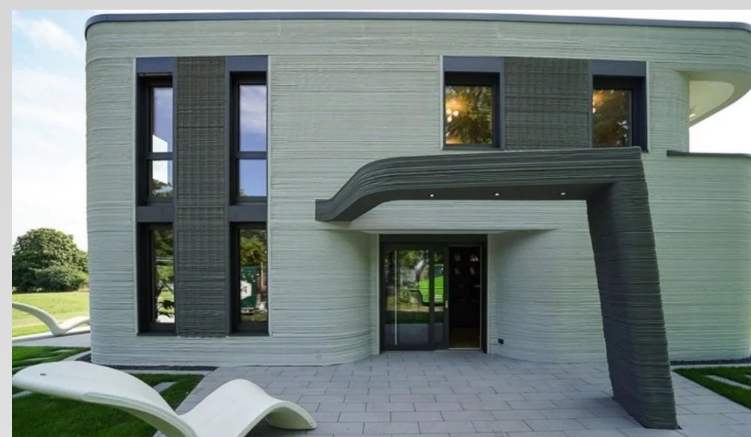
3D Printed House Constructed in Germany
